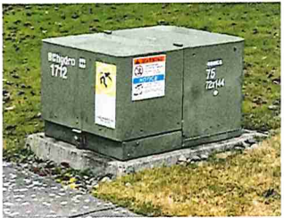
Pad Mount Transformer (PMT)
